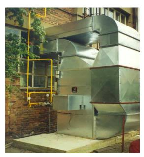
Centrifugal fan (event. double centrifugal fan) is situated in the frame of the unit just before the combustion chamber. Units can be delivered in designs with high-temperature or ventilation bypass that are
